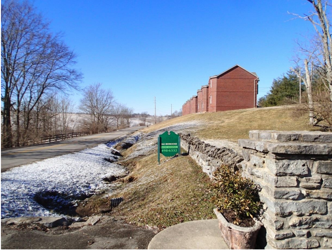
Figure 4-9. Sloped Area and Apartments, Looking West.
